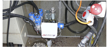
2013: The very compact CSV combination shaft valve is developed especially for use with NESSy and SnoTek guns.
